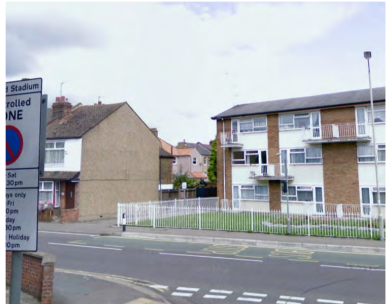
8 Existing vehicular access to the rear parking court and garages
