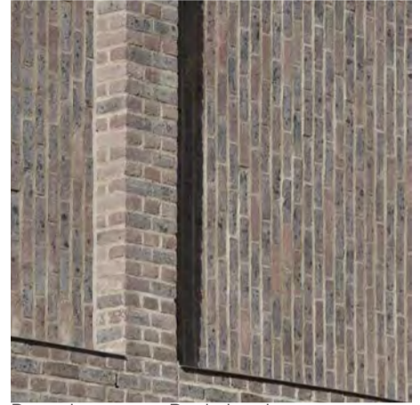
Precedent image: Brick detailing
