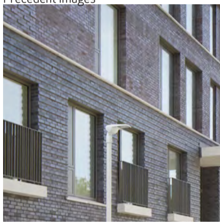
Protruding Brick Bands
