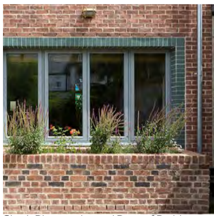
Shrub Planting Around Base of Building
