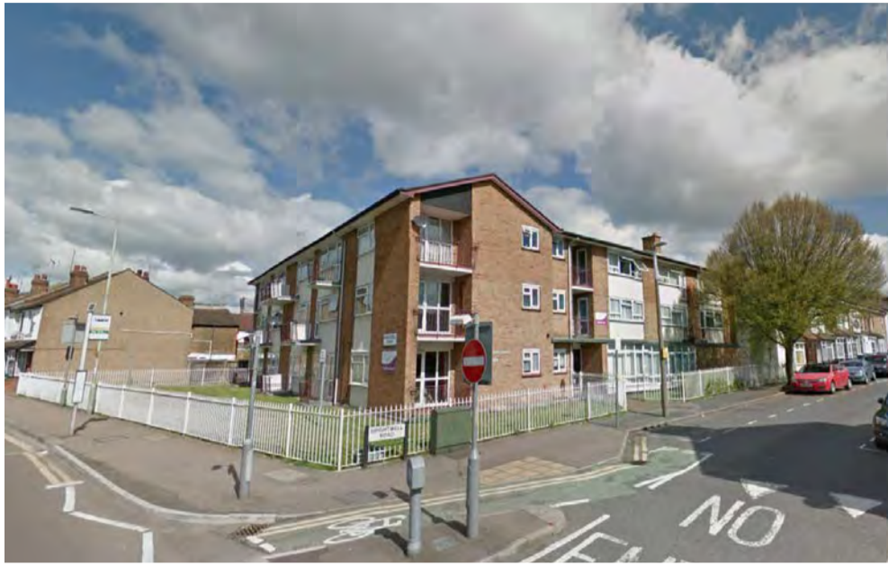
1 Brightwell Court from the corner of Hagden Lane and Brightwell Road. The exposed gable of a Hagden Lane terrace stands out as the building line of the existing steps back.
